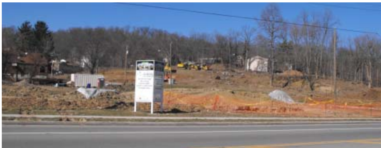
Clearing taking place for Virginia Place, Virginia Avenue just off Colerain
