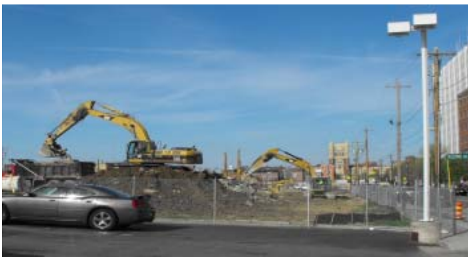
Work on site just west of Shell Station
